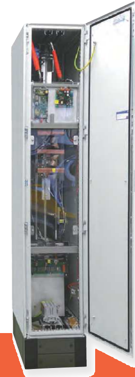
Hollow rope testing with 5000A
